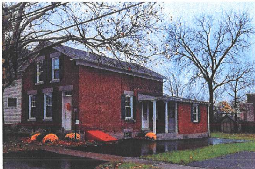
South Long Street elevation from the north, November 2022
