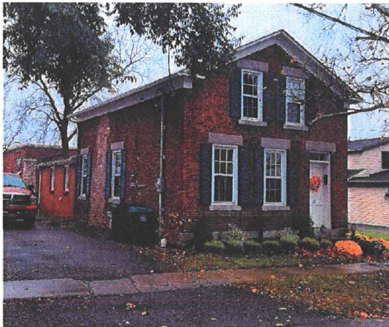
South Long Street elevation from south, November 2022
