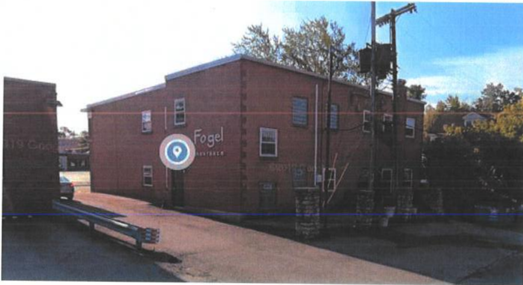
Figure 5: North and west facades from rear parking lot
