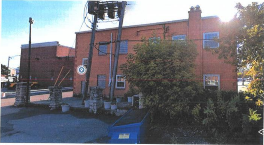
Figure 6: West façade with masonry patio and pillars, 2025
